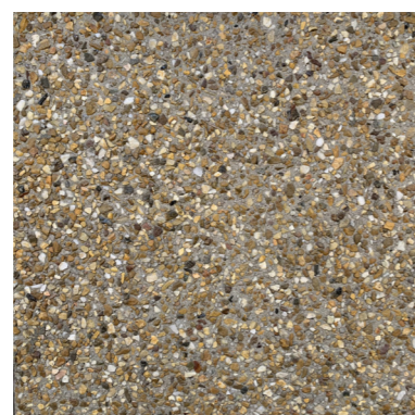
Exposed Aggregate Concrete
